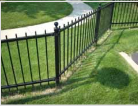
The perimeter fence that runs along the property line between the two developments is the responsibility of the Association
