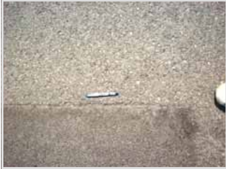
We recommend an annual review of the asphalt in the spring.
