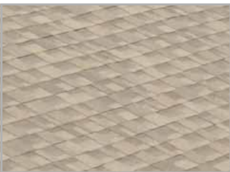
Basic maintenance is important to extend the life of the roofing
