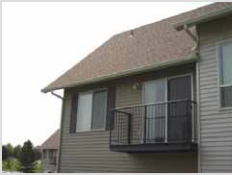
Replacement of the current roof is scheduled for 2026.
